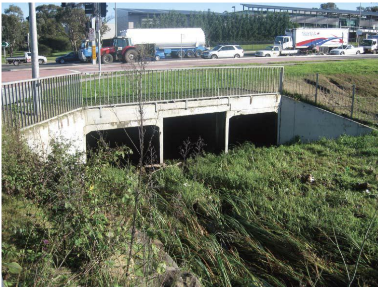
Figure 4. View of drainage culvert under Sunnyholt Road
